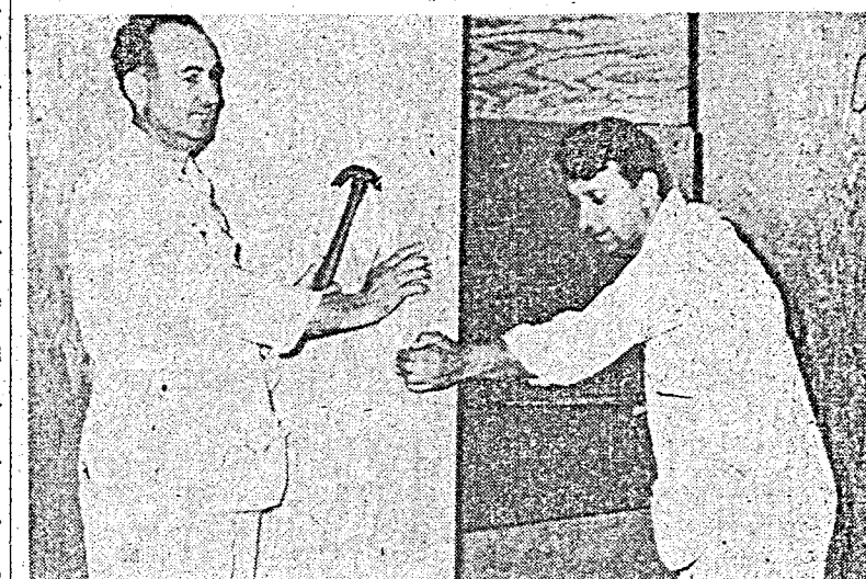
REMODELING—James Johnson (left), joiner, and James Bidolli, carpenter, Public Works maintenance branch, are shown putting up partitions to convert the Building 4 conference room into office space.
