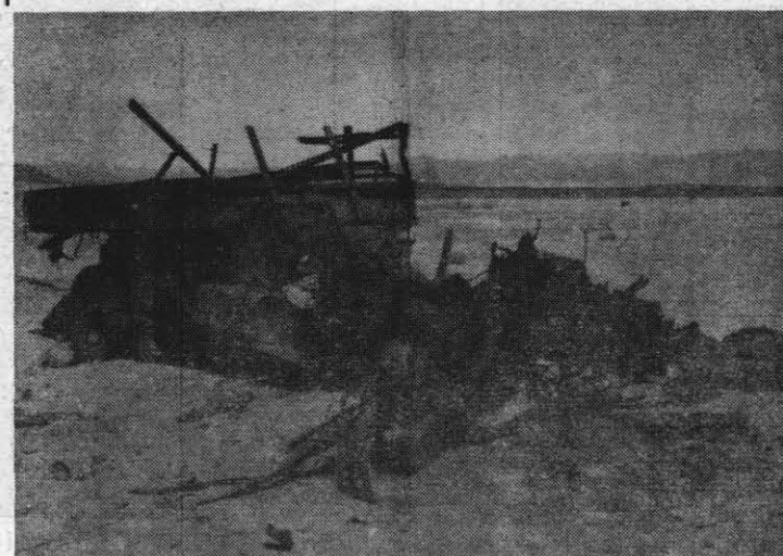
DRAMATIC evidence lies in wake of test drop of Snakeye weapon. Significant aspect of retardation device is elimination of fragmentation hazard to planes and reduction of skip tendency of bombs.
