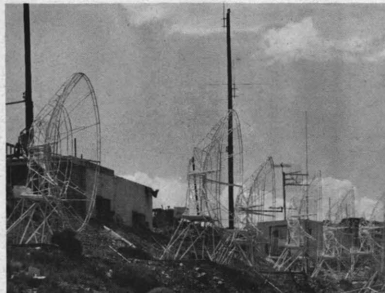
LAUREL MOUNTAIN is locale of tall tower under construction by Public Works Department for U.S. Air Force. Ninety-foot utility poles jut in the air to form base for test structure. Scope of Public Works ranges from design and construction of technical facilities to improving livability of China Lake community's living facilities.
