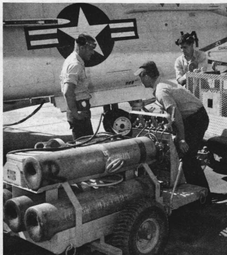
FILL 'ER UP BUDDY — Proficiency and a dedication to duty provides the motive for these airmen to give their A7A "tender loving care," keeping their aircraft in an "always ready" condition. Here, the VX-5 professionals are refilling air cylinders inside the aircraft.
