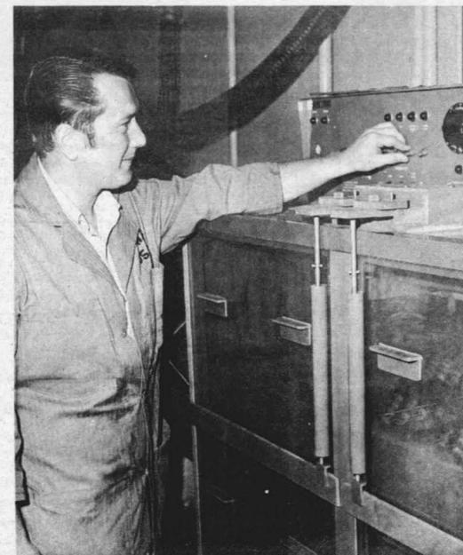
**SPRAY ETCHING**—Charles Knowles is shown adjusting the controls of an oscillating spray etcher. The machine sprays hot ferric chloride acid on the board as it is carried through the chamber on a conveyor. Rollers of the conveyor are visible through the clear polyvinyl chloride window of the etching chamber.
