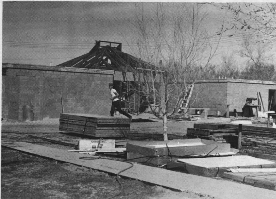
RECREATION AREA IMPROVED —Getting ready for the warm weather season, improvement work that is being carried out as part of the Navy Self-Help Program at the Naval Air Facility swimming pool is now nearly complete. Concrete block structures housing men's and women's shower and restroom facilities, and separated by a shaded snack bar in center, have been built with the help of four SeaBees and the volunteer aid of a group of around 10 enlisted men from NAF. Another SeaBee enlisted man is scheduled to report to China Lake this week and, joining the others already on board, will begin remodeling work at the NWC Enlisted Personnel Barracks (No. 880), where three wings are to be converted from cubicles to rooms.
