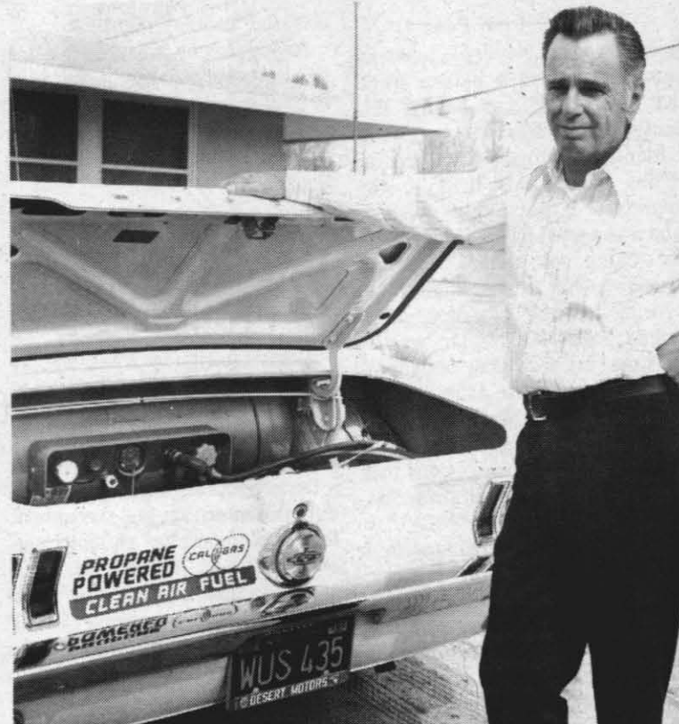
NON-POLLUTER —The trunk of Jack Richards' 1968 Mustang encloses a special fuel tank containing propane (liquefied petroleum) gas. Unhappy over the way gasoline caused carbon to foul up the engine of his car, which he uses mainly for low-speed driving in the local area, Richards had his machine modified to use PL gas for fuel.
