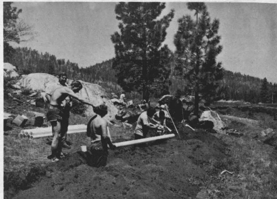
SEABEES ASSIST BOY SCOUTS — Members of the RMCB 0417, Las Vegas, Nev., and the locally-based RMCB 0217 are shown laying a section of 700 feet of plastic water line at Camp Nick Williams on Piute Mt. The Seabee Reservists spent a day at the Boy Scout Camp digging the trench, blasting through rock formations (with the assistance of the NWC EOD Office), installing a gate and surfacing the swimming pool at the camp.
