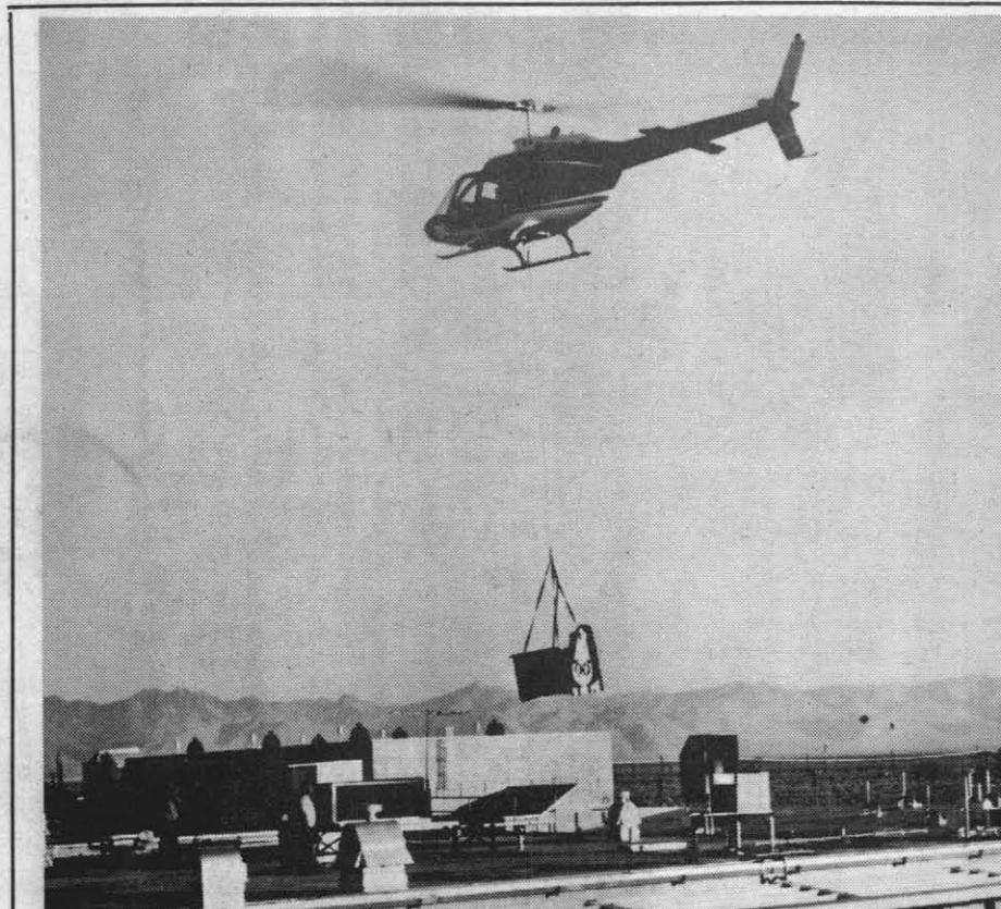
BIG MOVE — A Bell Ranger helicopter, owned by the Briles Fixed Wing and Helicopter Co., is shown moving one of three sections of a 1,900-lb. air conditioning unit to the top of Michelson Laboratory. The big lift, which was accomplished at 6 o'clock on the morning of June 5, saved many man hours and was closely observed by many NWC construction personnel.
