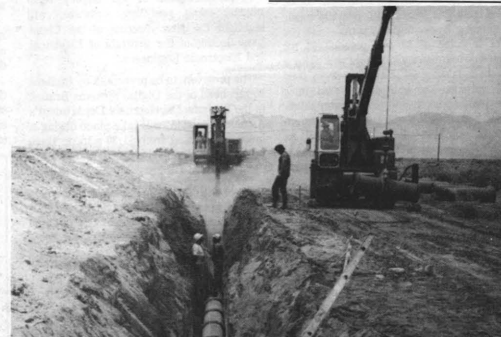
SEWAGE LINES INSTALLED — Workmen for the Wal Con Construction Corp. of Sherman Oaks, Calif., are shown installing a section of 15-in. sewer line that will extend from the sewage treatment plant at China Lake to connect with an existing line just north of the Ridgecrest Community Hospital. In addition to the installation of a larger (27-in.) sewer main that is to be laid just east of Richmond Rd., plans also call for increasing the capacity of the China Lake sewage treatment plant in order to meet the anticipated needs of the local area for the next 20 years. —Photo by Peter Anders
