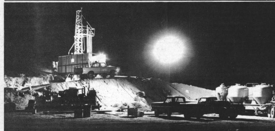
**NIGHT OPERATIONS NECESSARY** — Two shifts are worked normally during drilling operations at the Coso geothermal area. However, once the drilling had reached the point where it was ready for cementing the casing, this job had to be continued until it was completed as the above photo (taken around midnight)
