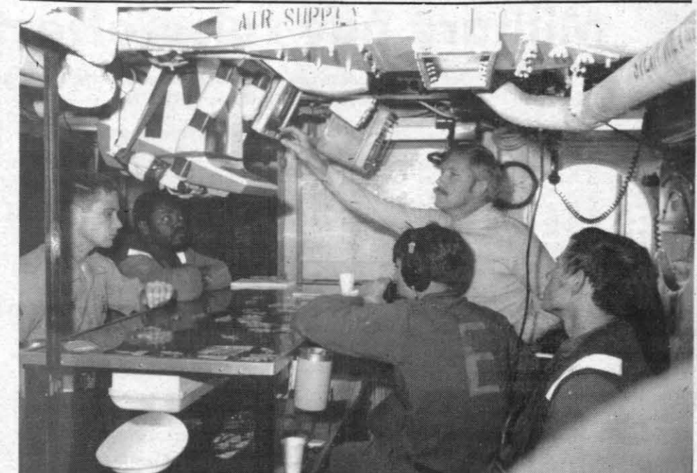
VITAL MISSION — LCDR Bud Morris, Kitty Hawk's handler, uses a television screen (called a PLAT) to observe the recovery of aircraft, and, to its left, a LINDA console to learn of the fuel, radio frequency, maintenance problems and other details of airborne aircraft. This is done from the flight deck control room, where enlisted personnel can be seen bending over the Oujia board, which displays the location of aircraft on flight and hangar decks.
