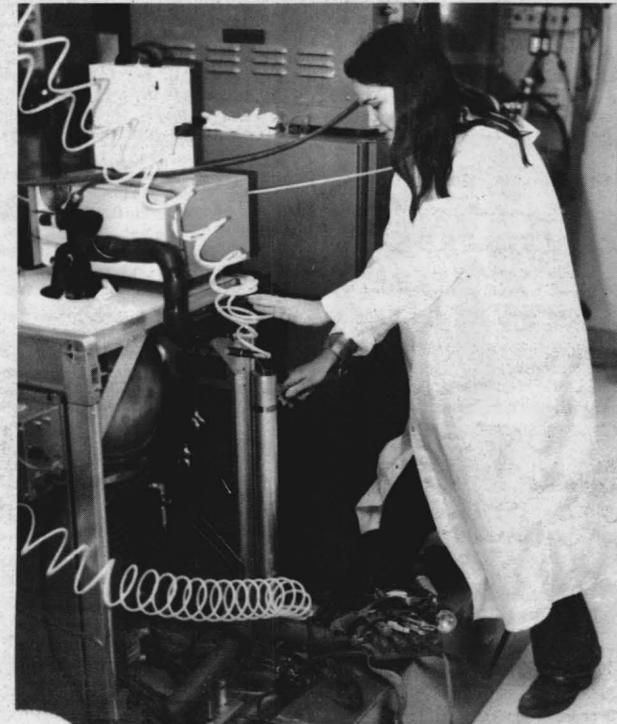
**EXAMPLE OF WORK** — Ann Stark, recently promoted from helper to intermediate journeyman status as an air conditioning equipment mechanic, works on modification to a thin film sputtering deposition system that is used in the microelectronics laboratory to apply specialized thin film coatings to substrates. She replaced a liquid nitrogen cooled cold trap by one that makes use of freon as a cooling agent. —Photo by Ron Allen
