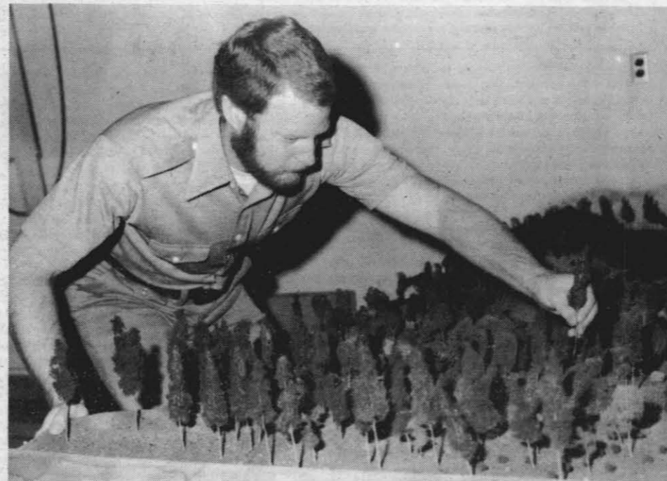
TREE PLANTING —Jeff Grossman "plants" a tree in the styrofoam-like base of the 1:84 scale terrain model used for testing the effectiveness of various types of camouflage of military vehicles. Discoveries made regarding effectiveness of various colors and patterns of paint on vehicles, and of the value of using fender skirts on tanks to disguise their configuration, were recently reported at a NATO working group conference in Germany. —Photo by Ron Allen
