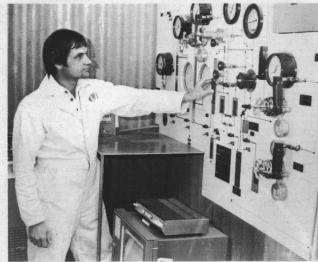
**GAS PRESSURE BOOSTED**—In the safety of the control room, Gary Smith, shown at the control panel of bench-scale pyrolysis gas purification and polymerization system, prepares to boost the pressure of purified gases before they go into the polymerizer.
