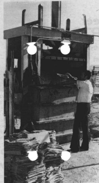
**BALING** — Newspapers collected are sorted (to remove cardboard or magazines) and then baled for ease in handling. As they are baled, they are sprinkled with water to help cut down on dust (up to 5 percent of weight of newspapers collected for resale can be water). Jim Fath gets set to toss a load in the baler.
