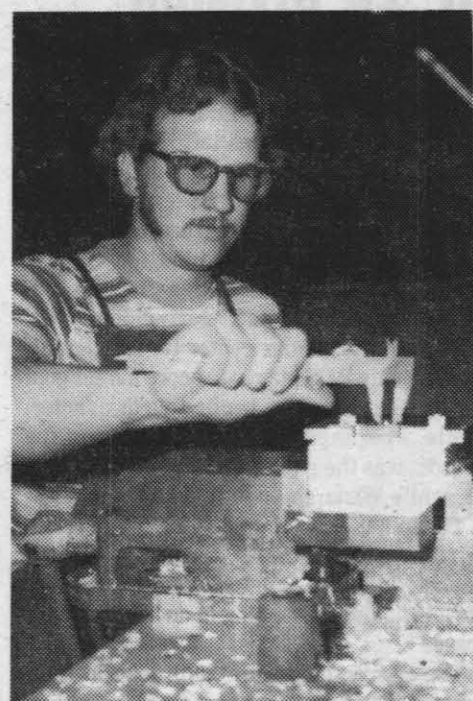
PRECISION WORK — Gary Ford, who recently completed prejourneyman training as a machine tool operator, finishes rings using a numerical controlled mill.
