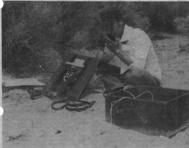
**SOUNDING STATION MANNED** — Stephen Waddell, crew manager for General Electro-magnetic Prospecting, Inc., measures different electrical frequencies as they come back through the ground. Data from this sounding station and others like it will provide a clue to the underground rock structure in the Coso geothermal area by indicating the resistivity of the earth. —Photos by Ron Allen
