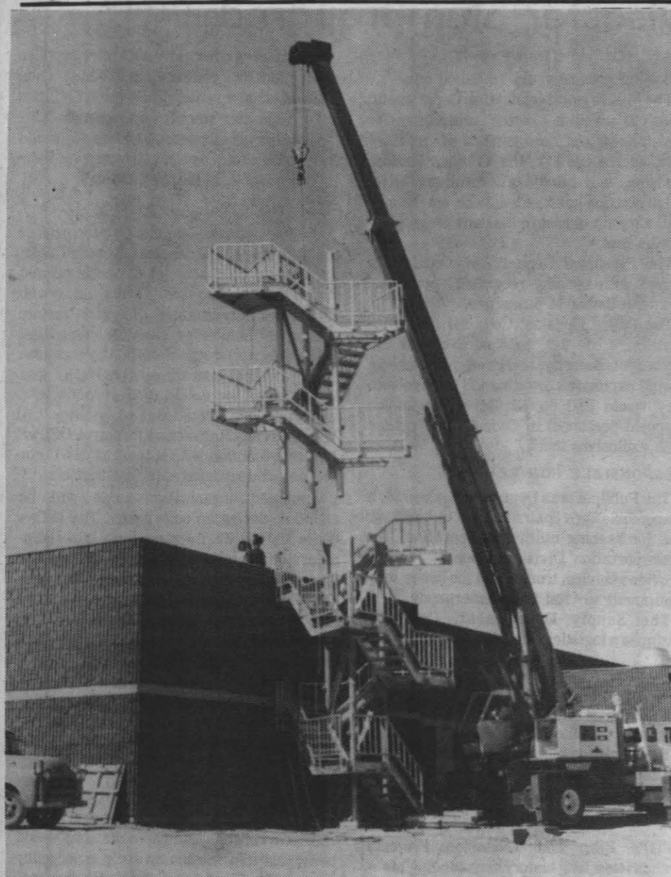
MICROWAVE TOWER ERECTED — A tower that will support a microwave tower goes up at the Range Control Center building, which is located east of Armitage Airfield at the intersection of Water Road and the range access road to Charlie Range. The microwave antennas will be fastened to hand railings for the staircase that will allow employees to climb to the top of the tower, which is 63 ft. tall. This building, which is the heart of the Naval Weapons Center's range improvement and modernization program, is approximately 85 percent complete. Contractor employees are involved in interior painting work, installing doors, and making some of the final electrical connections.
