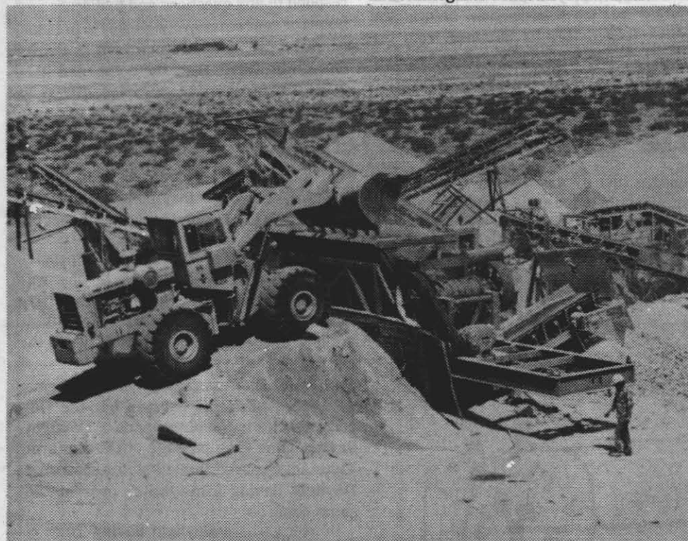
GRANITE CRUSHED FOR RUNWAY PAVING — A batch plant and crusher operation has been set up near B Mt. by Desert Construction of Victorville, the successful bidder on a $750,000 contract to resurface the main runway (3-21) at Armitage Airfield. Two 8-hour shifts are now being operated to convert the native granite rock material for use as part of a 2-in. overlay of paving material on the 200 ft. wide runway. The job calls for heat scarifying the old runway surface, applying a rejuvenating agent, and then installing the new paving.
