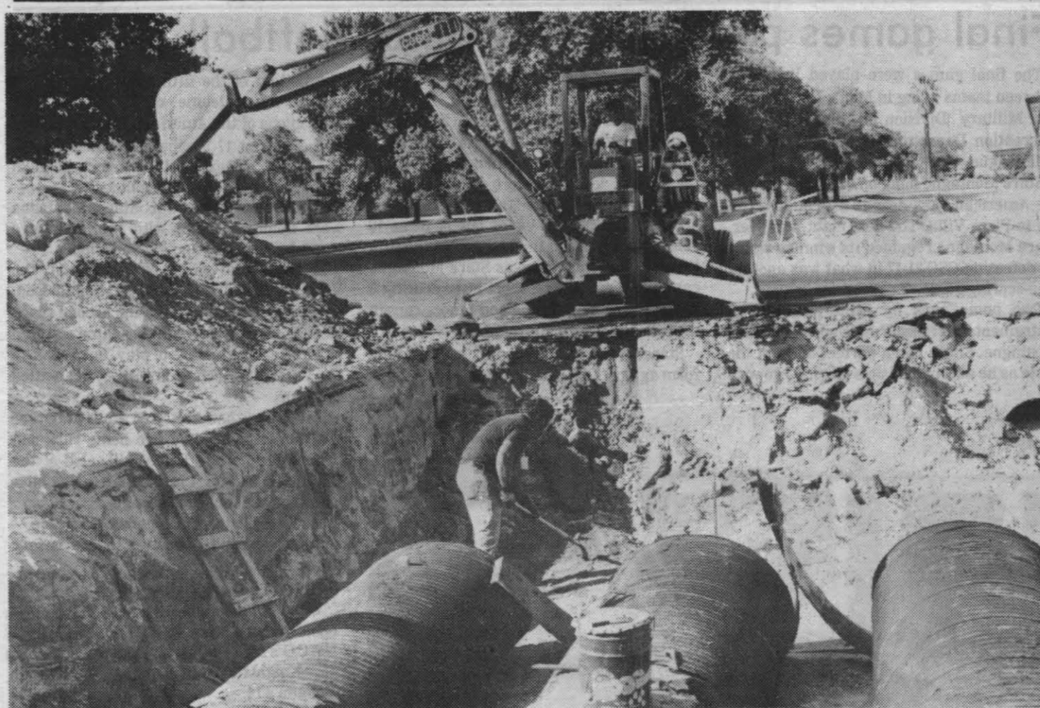
DRAINAGE SYSTEM IMPROVED — Workmen for the James W. Ford Co. of San Bernardino are busy with the task of regrading drainage channels and installing new drainage pipe along Knox Road from a point just south of Blandy Avenue north to the vicinity of the sewage disposal area ponds. A contract for this
