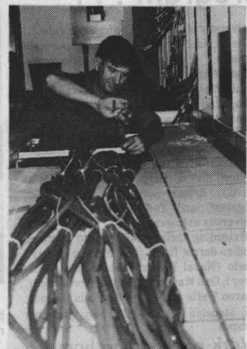
CABLES APLENTY — Army S/Sgt. Dwayne Dickerson prepares to install cables that are placed beneath the floor of the Range Control Center's Video Operations Center.
