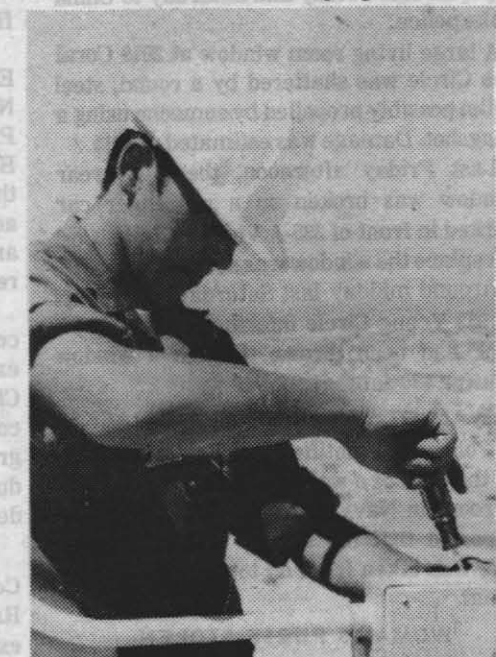
WORKS ON ANTENNA — Army Spec. 4 Daryl Jones, who is completing the installation of an antenna at the top of the tower, is a member of the team headed by Sgt. 1st Class Joseph Radosevich that is involved in installing microwave, UHF and VHF antennas on the RCC's 65 ft. tower.
