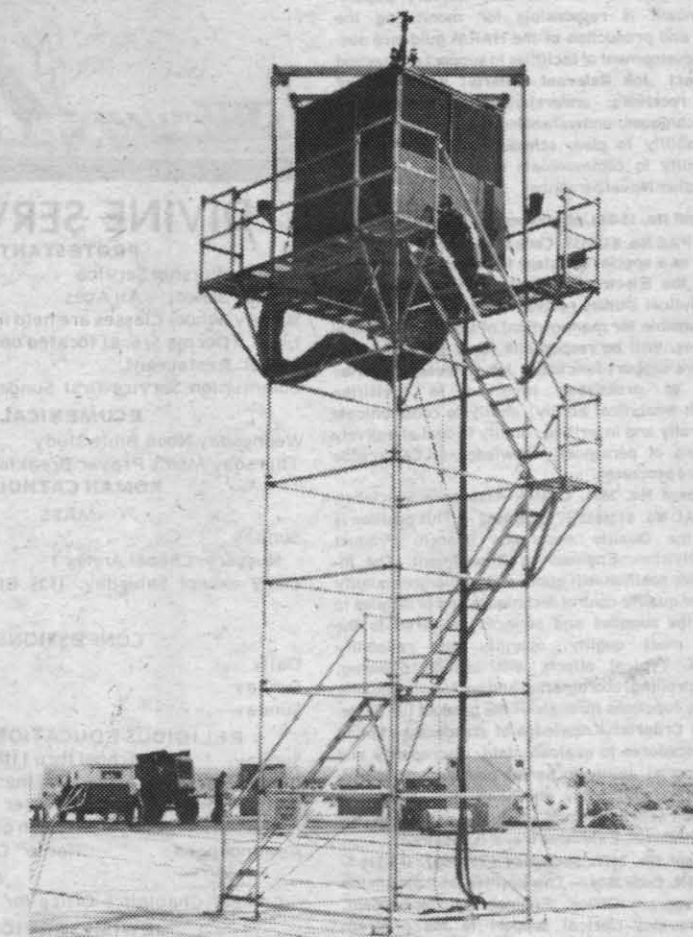
TEMPORARY TOWER — This prefabricated portable air traffic control tower located in the gun butts area of Armitage Airfield serves as the Center's air traffic control tower while the permanent facility is being renovated and new equipment installed.
