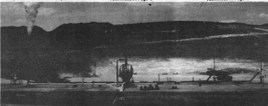
**CURRENT PHASE OF TEST WORK** — Tests to determine the characteristics and productivity of the underground reservoir of steam in that portion of the Coso Known Geothermal Area where test wells have been drilled are expected to be completed by this weekend. A test array that separates steam from water is currently set up on the third drill pad. Dick Adams is in charge of the reservoir
