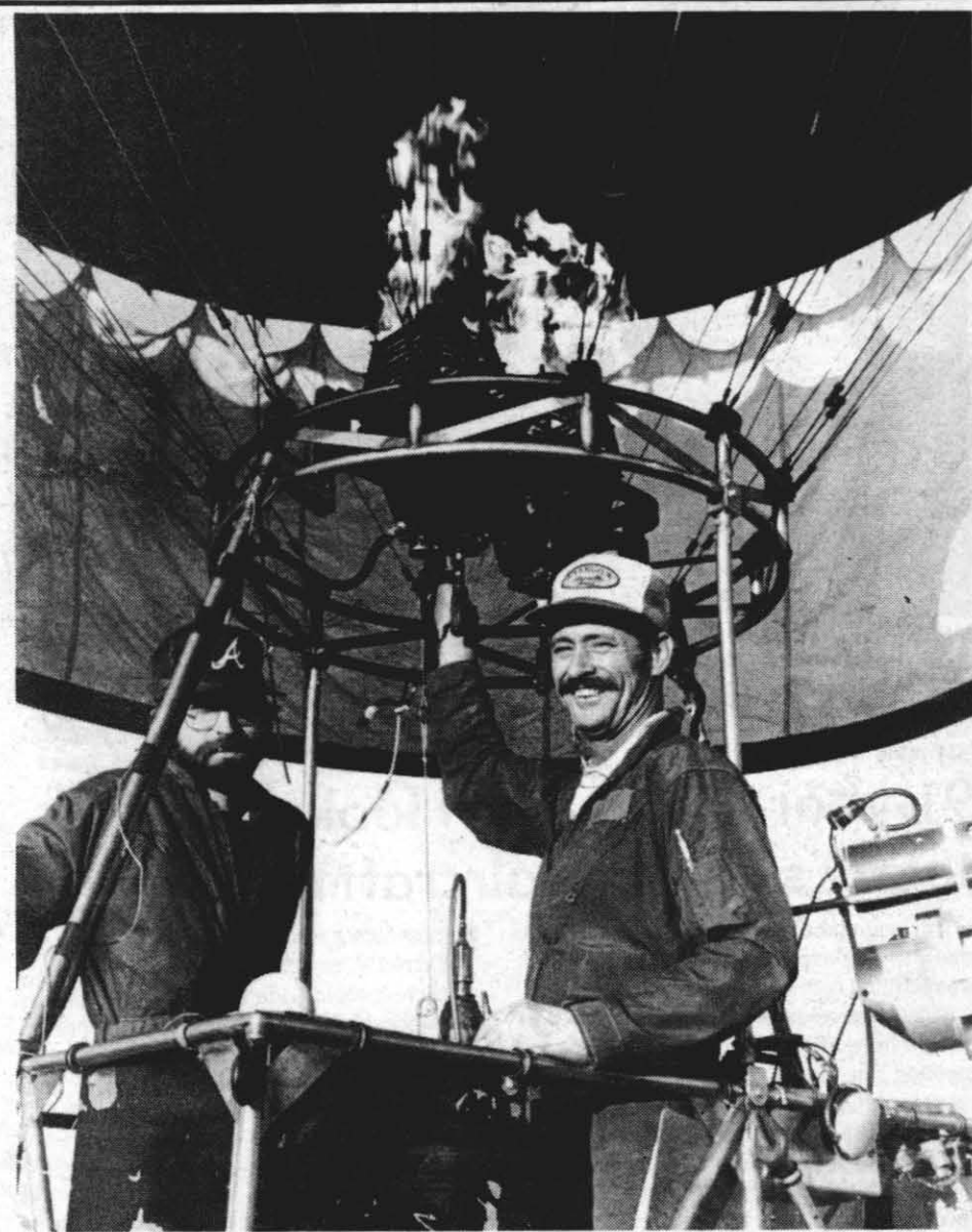
FIRING UP — Art Hickie, who is in training to handle balloon test flights, watches as Duane Powers, the Center's Chief Balloonist, tweaks the propane burners used to produce the hot air needed to fill the balloon. — Photo by Jerry Morrison
