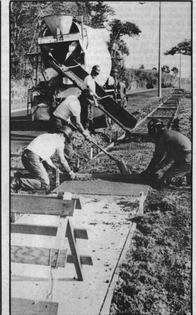
SIDEWALK WORKERS — Real sidewalk superintendents, Seabees use their concrete construction skills to put in a sidewalk. Workers on the project included (from left) CM3 A. W. Brogdan, BU2 B. Vargus, CE2 C. R. Allen and CE2 R. M. Gil.
