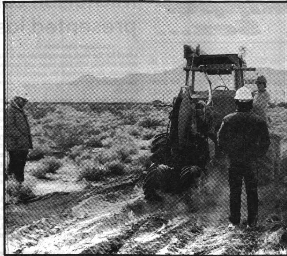
FOTS WORK —Employees of Kendall Telephone Contracting Co. lay fiber optic cable between Armitage Field and SNORT as part of the Fiber Optic Trunk System contract at NWC.
