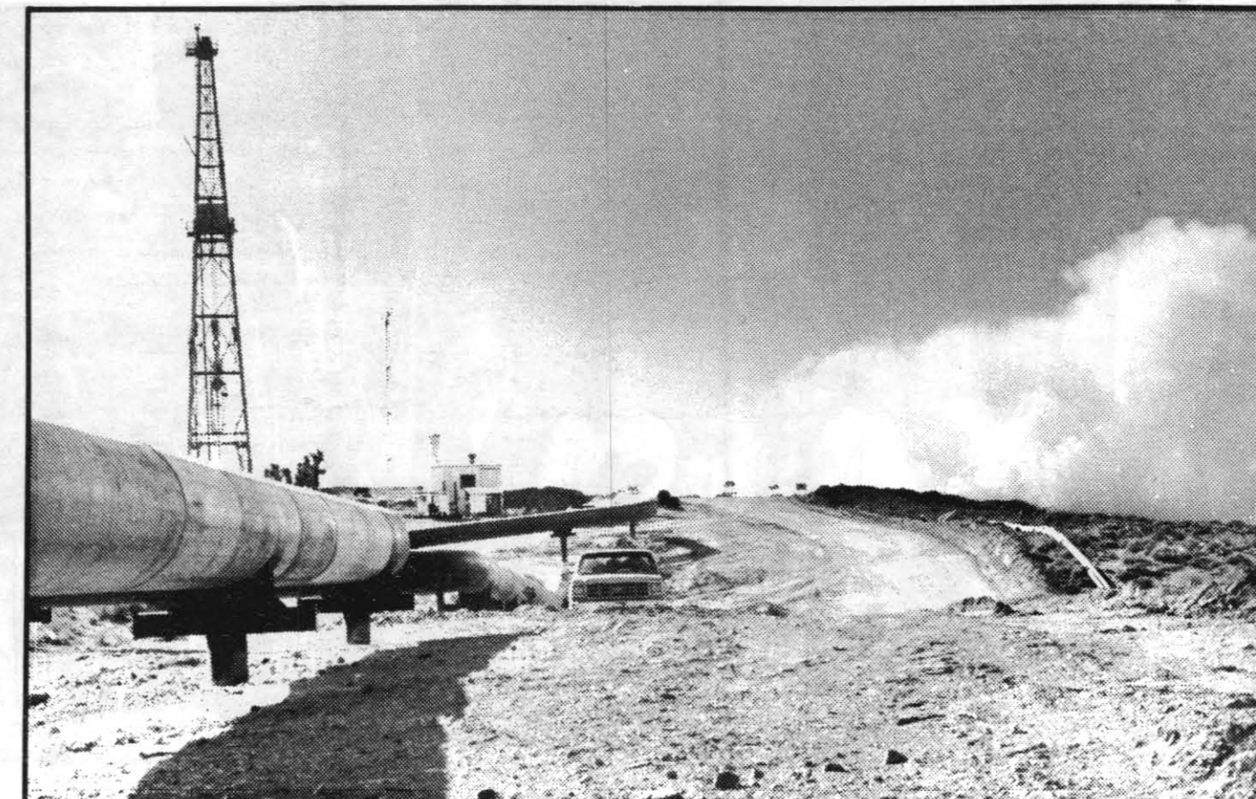
NEW WELL — Drilling for a new production well at the Coso Site is well underway. The drilling rig is framed by the pipeline that will carry geothermal steam to the power plant and clouds of steam generated by the drilling process.
